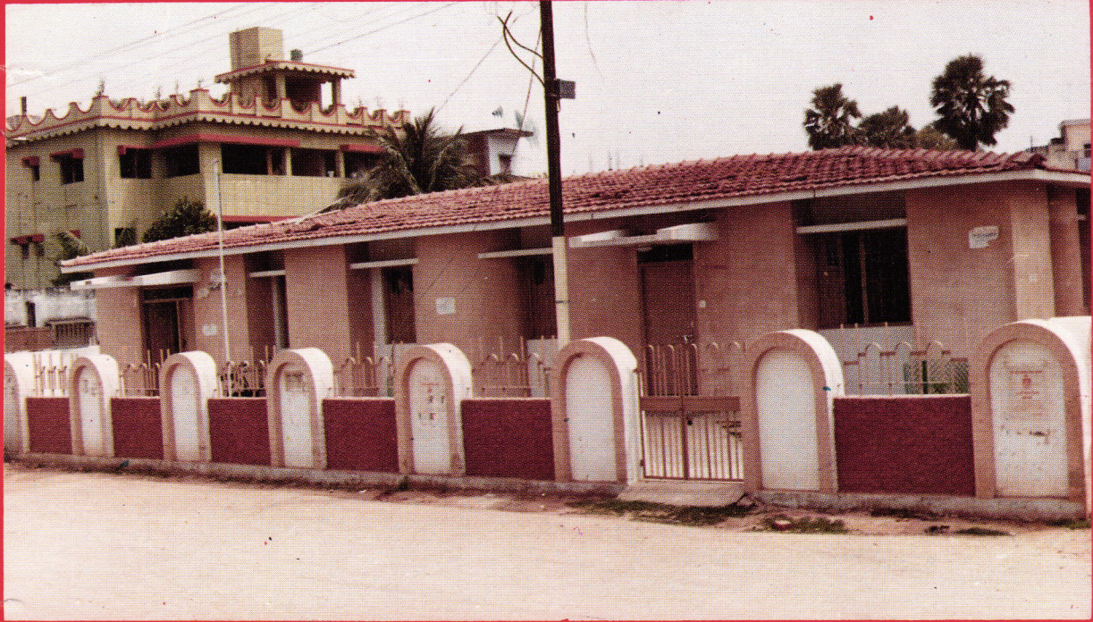
Kidwaipuri Post Office Building, Patna
