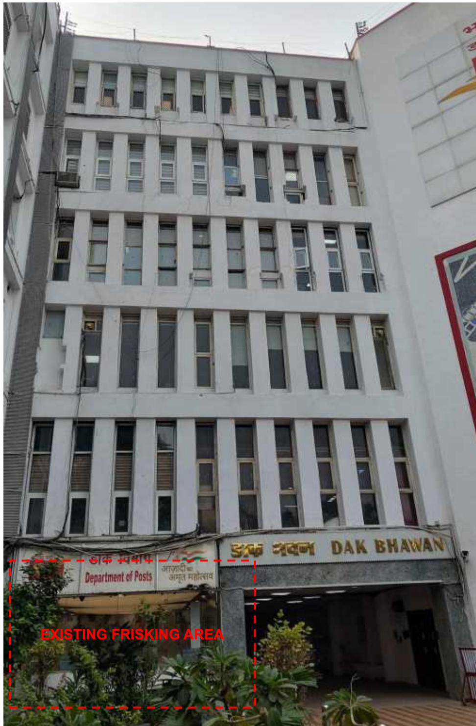
Image 30 : Existing facade near reception. (Source-Author)
