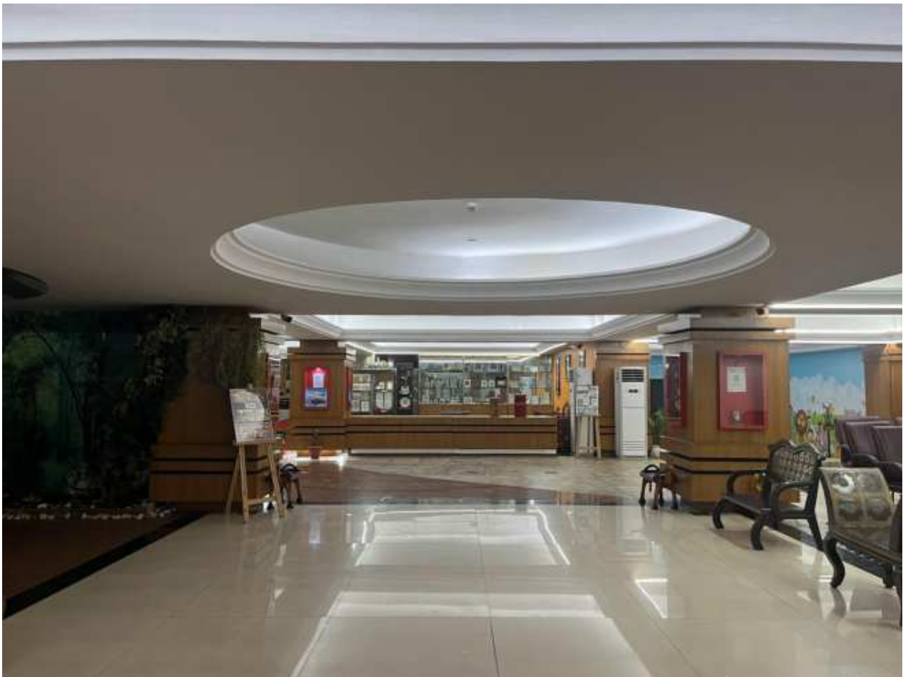
Image 17 : Interior of existing Philatelic Museum. The floor is punctuated using various materials in geometric shapes creating visual separation. The ceiling includes recessed geometric shapes like circles and rectangles. The walls/columns are treated in veneer finish. (Source-Author)
