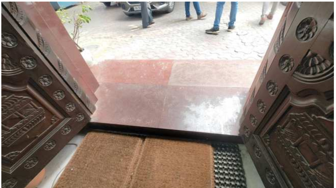
Image 32 : Floor level difference at museum entry. (Source-Author)
